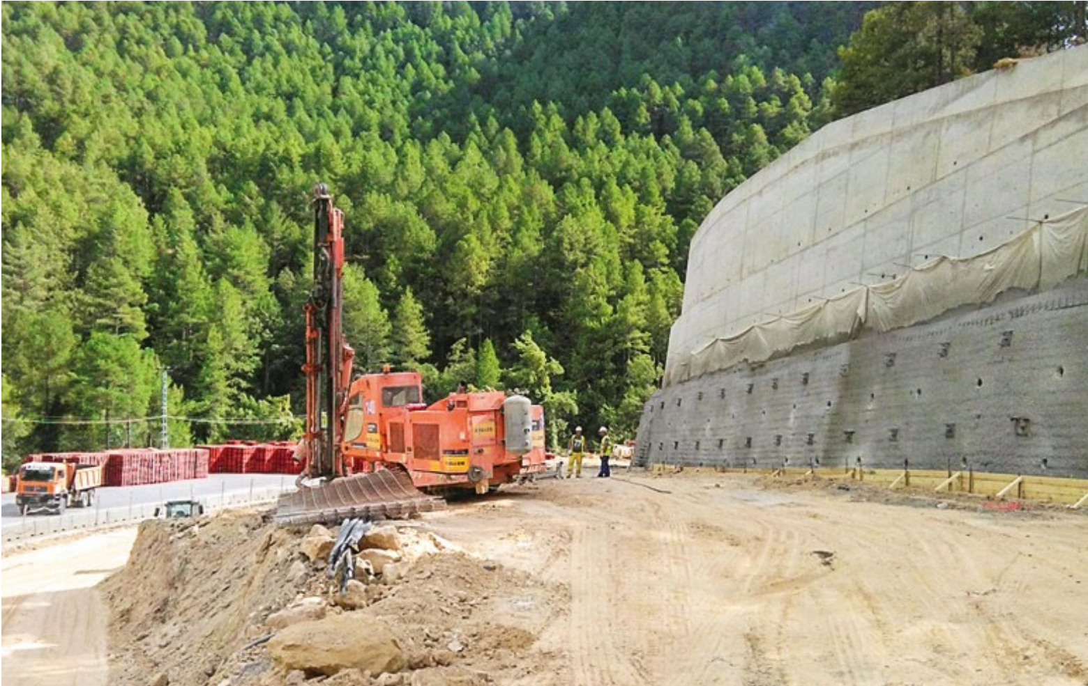
Photo reprinted courtesy of Keller Cimentaciones, S.L.U., Spain
