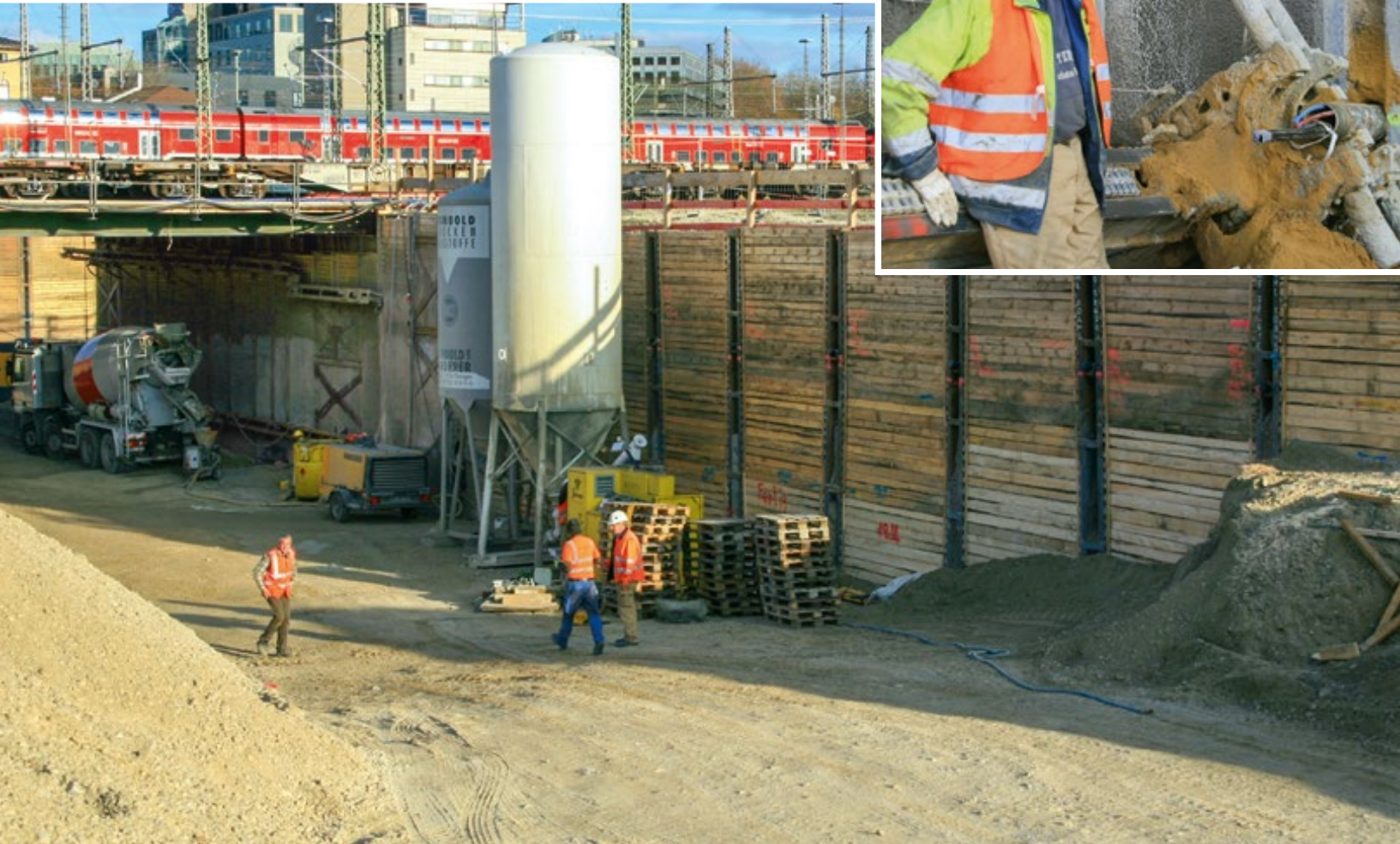
Photos reprinted courtesy of Stump Spezialtiefbau GmbH, Germany
