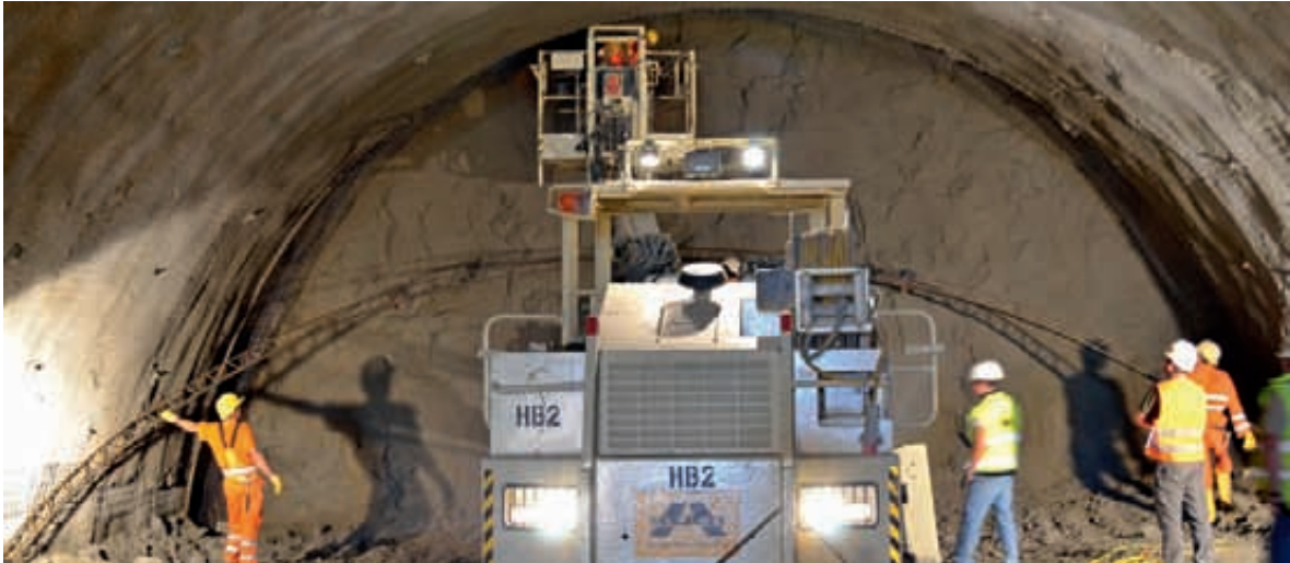
Photos reprinted courtesy of Alpine BeMo Tunneling GmbH, Austria
