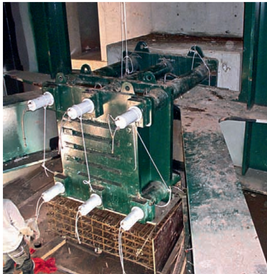
Preparation of Wax Injection into the Ducts
