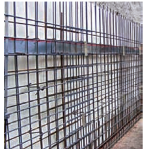
Preprufe® Sealing Strip in the Wall Area with additional contaflexactiv Joint
