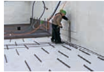
Preprufe® – the Sealing Strip System for unset Concrete with Approval for Sealing Surfaces.
