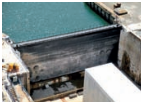
New Lock Gate
