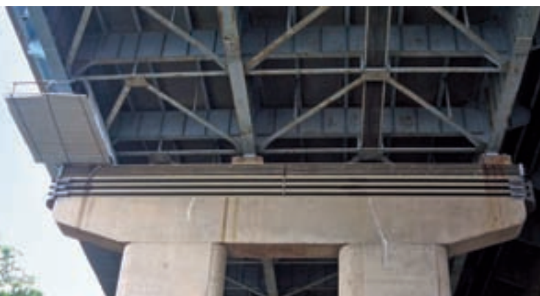
External DCP Bars with DYNA Force® Sensors
