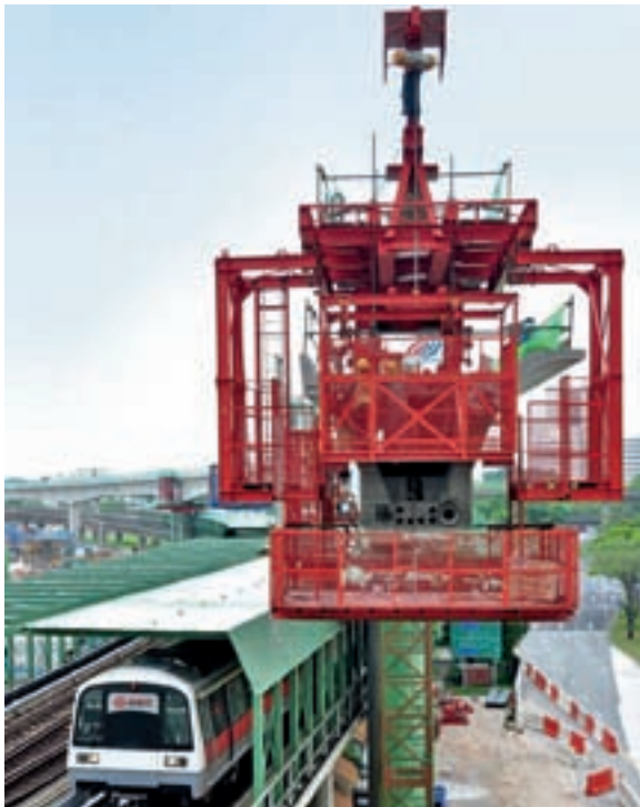
Viaduct spanning across a Railway Line in Operation
