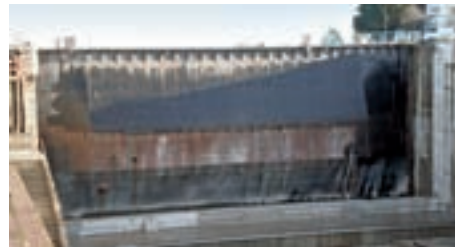
Dry Dock with old Lock Gate
