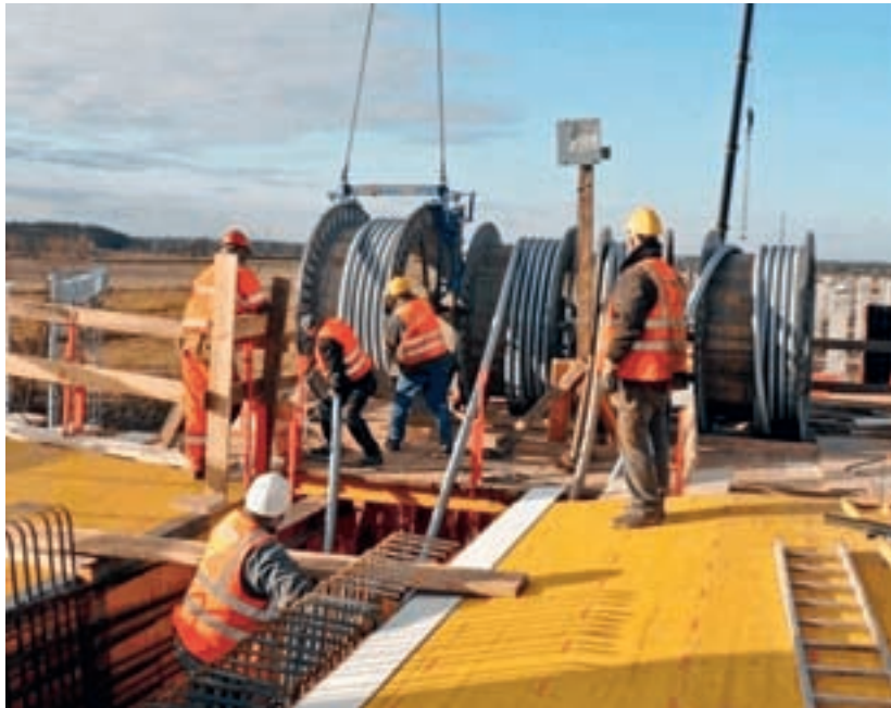
Uncoiling of Prefabricated Tendons and Installation in the Formwork
