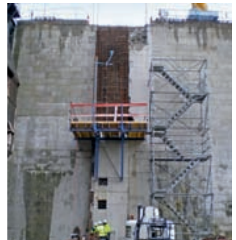
Reinforcement of the Outer Walls for the new Lock Gate
