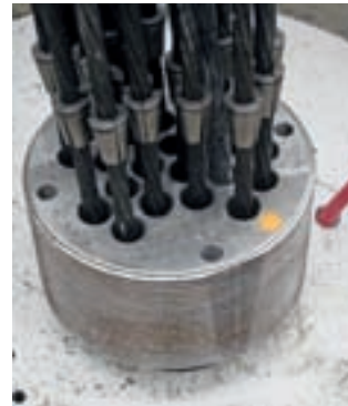
Wedge Plate for Restressable 20 Strand DYWIDAG Anchors
