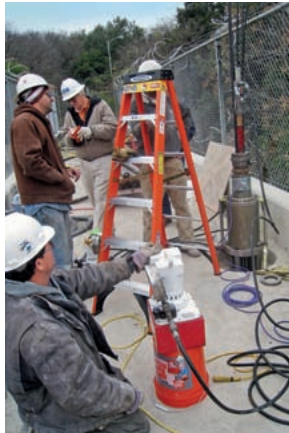
Alignment and Stressing of Six Strand DYWIDAG Anchors
