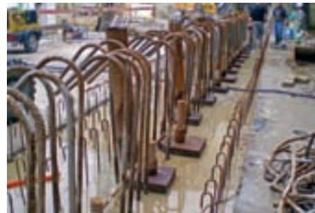
Installed DYWIDAG Bar Anchors
