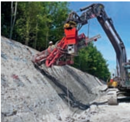
Excavator with Drill Boom
