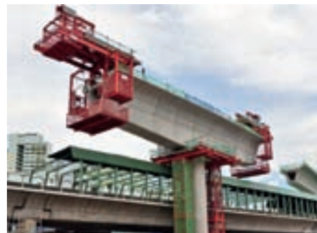
Working above a Railway Line in Operation
