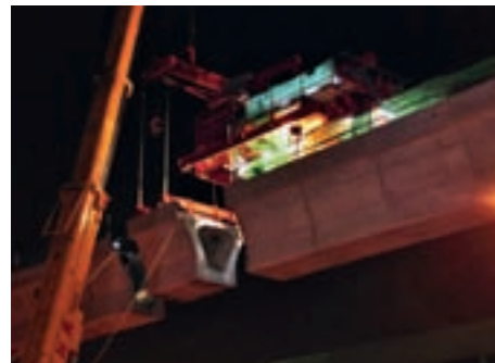
Launching of a Segment
