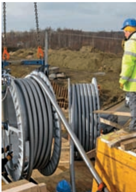
Prefabricated Type SUSPA Systems Tendons on a Drum
