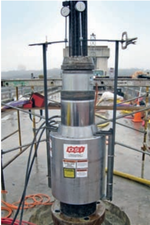
Stressing 20 Strand DYWIDAG Anchors with Tensa 6,800 Jack
