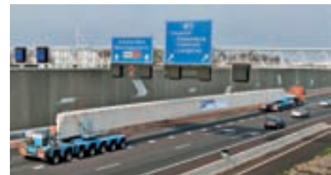
Transport of the Girder
