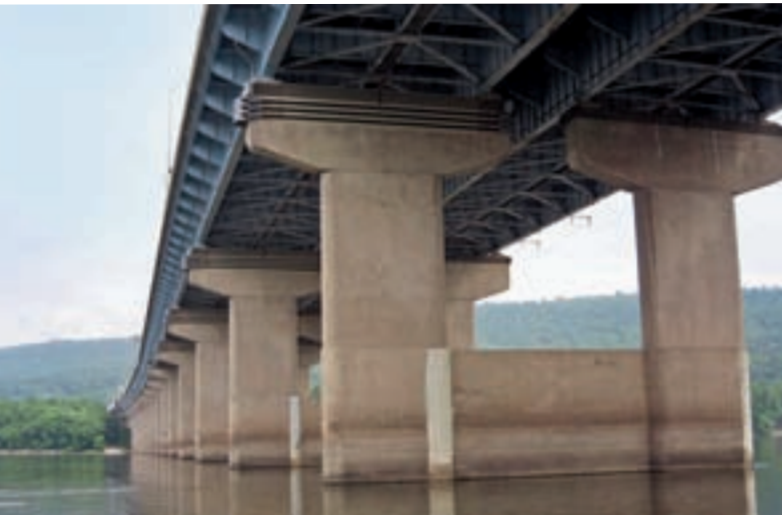
External DCP Pier Cap Strengthening
