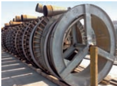
Prefabricated Type SUSPA Systems Tendons on a Drum
