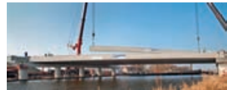
Placing the Box Girders
