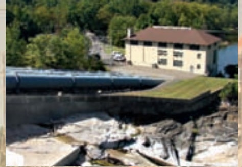
Penstocks with turbine house
