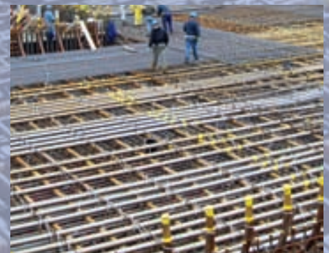
Horizontal Ducts for DYWIDAG Post-Tensioning Tendons in the bottom slab
