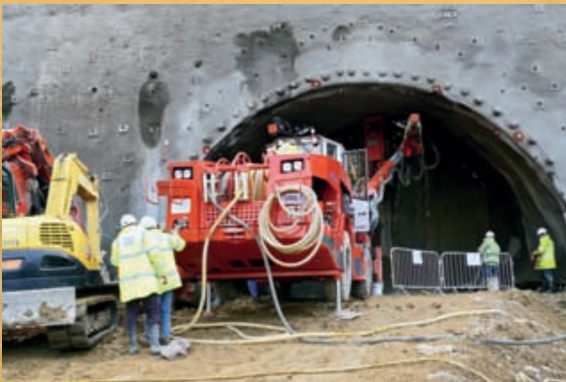
North Portal Tamrock Axera 8
