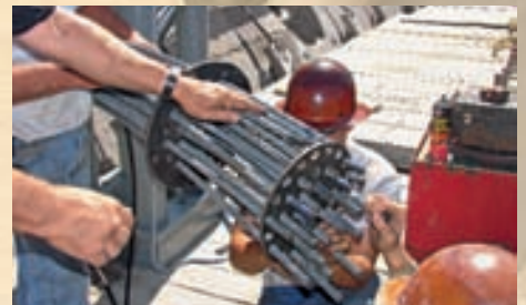
DYWIDAG Multistrand Anchors before Tensioning
