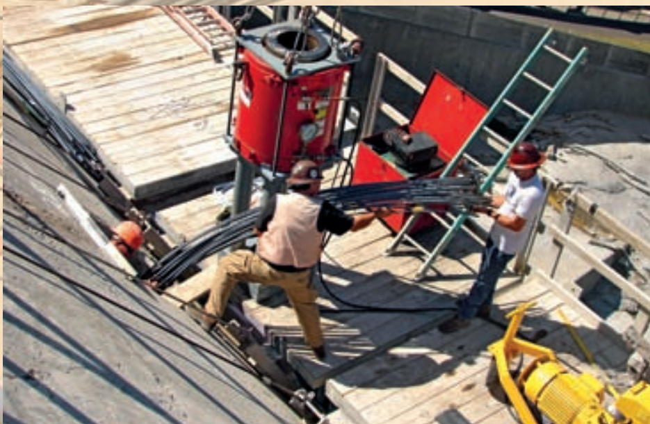
Installation of DYWIDAG Multistrand Anchors below the crest into the dam
