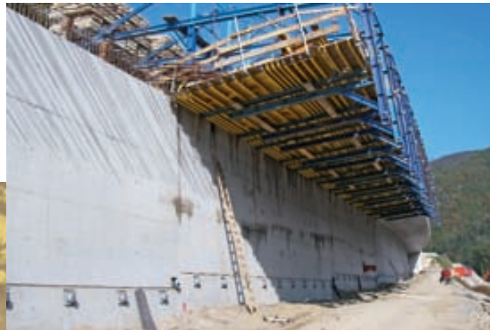
Finished anchor heads
