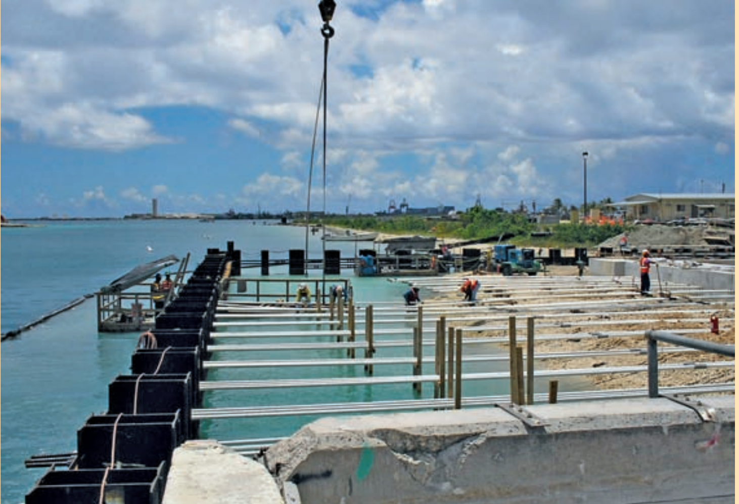
Tie Rod installation
