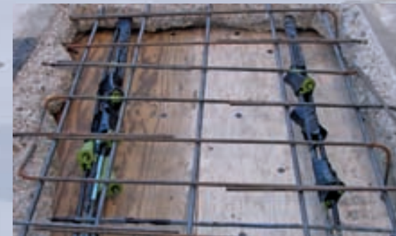
Ends of tendons waiting to be linked with couplers
