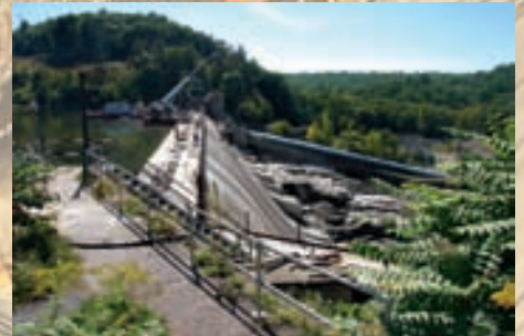
Overview of the dam
