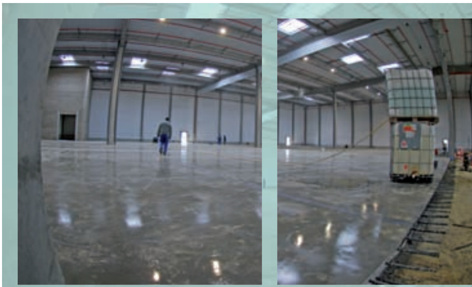
Utilization of Protecdal during concreting
