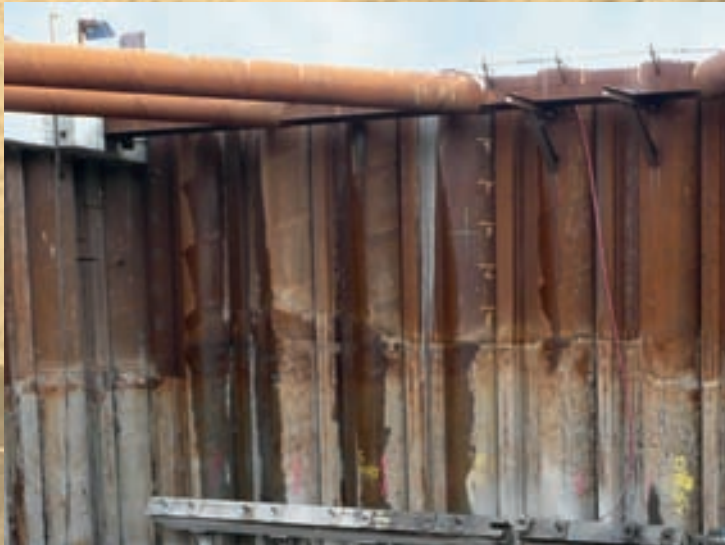
North Side float out structure
