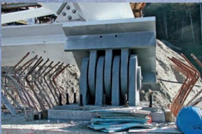
Installation of pivotal bearing
