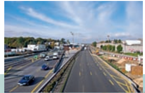
Overview of overhead noise barrier on motorway A86 near Paris
