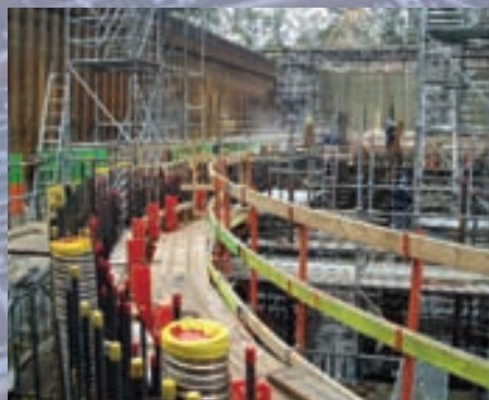
Vertical Ducts for Post-Tensioning in Walls
