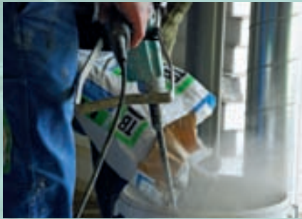
Utilization of Ravalchoc AL (powder with resin) for floor levelling
