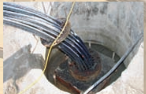
DYWIDAG Multistrand Anchors before Tensioning
