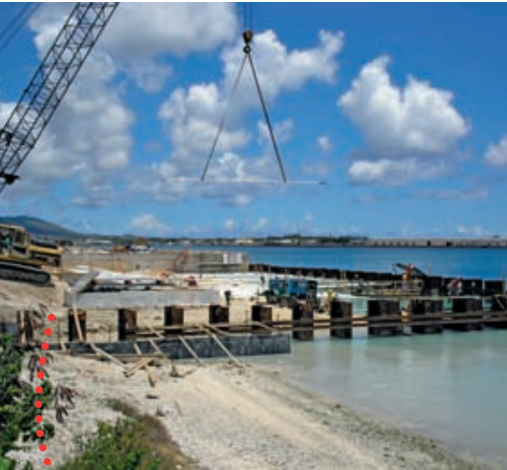
Levying of Tie Rods
