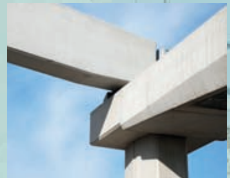
Detailed view of bearing profile with beams
