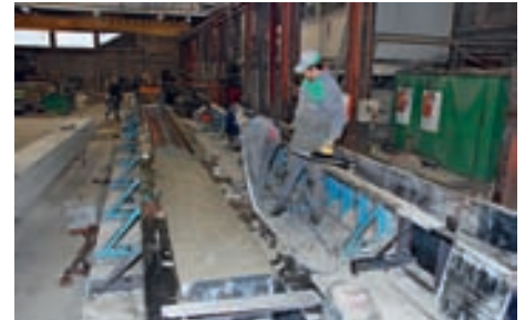
Concreting and formworking
