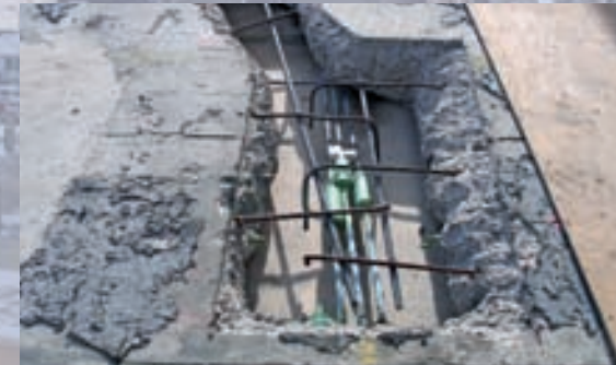
Monostrands with reinforcement before concreting
