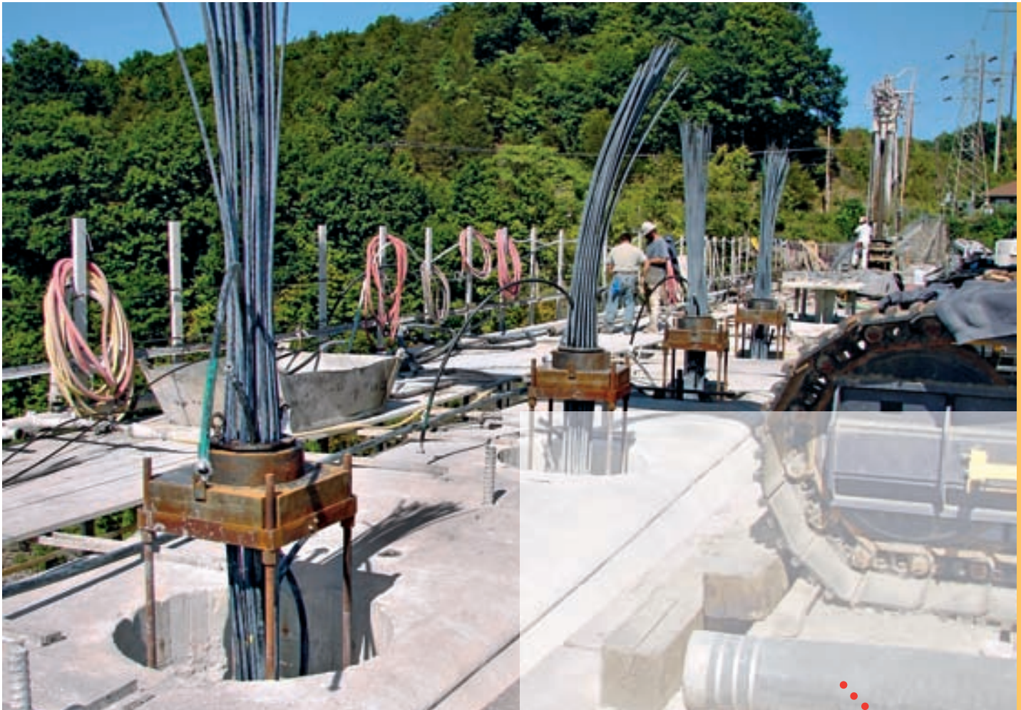
Installation of DYWIDAG Multistrand Anchors in the crest
