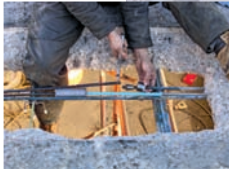
Installation of coupler splices
