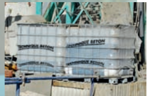
Concrete mixing facility with superplasticizer Addifor 2001
