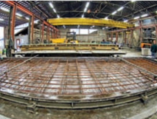
View of production facility
