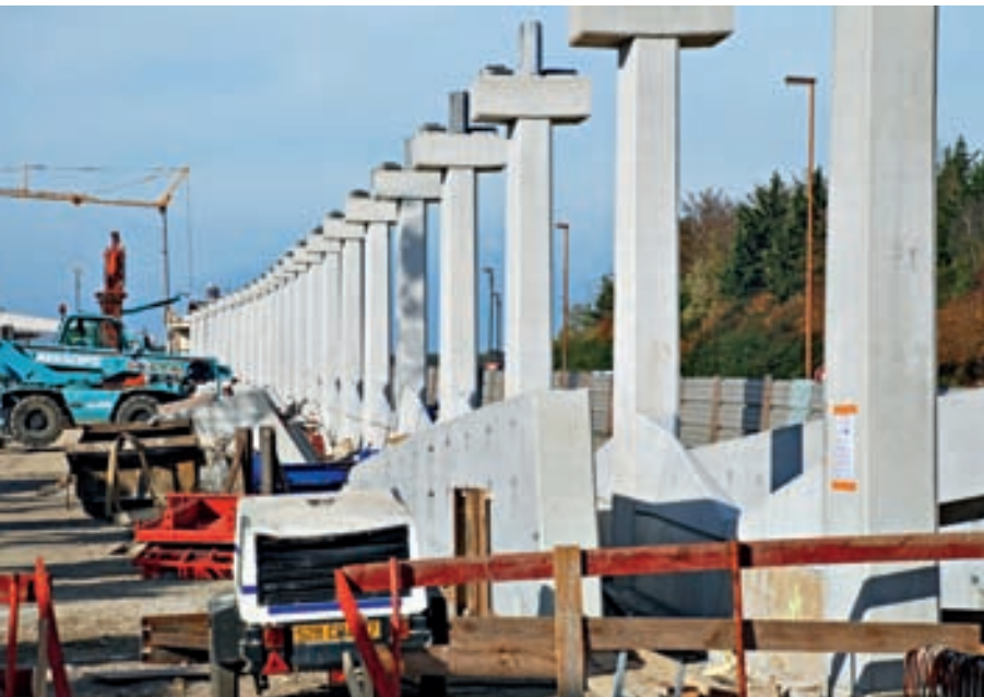
Construction of the high quality smooth bearing profiles
