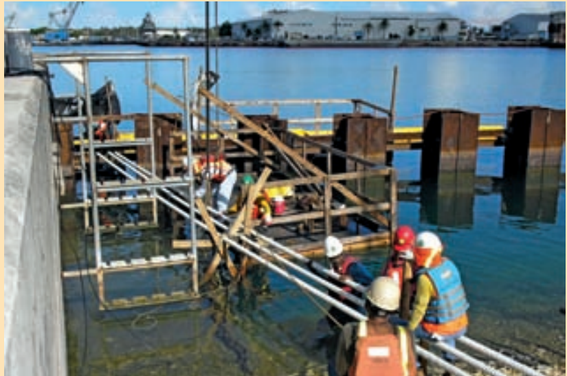
Installation of Tie Rods at sheet piles
