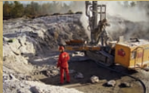
Boring of anchorage boreholes into the granite rock
