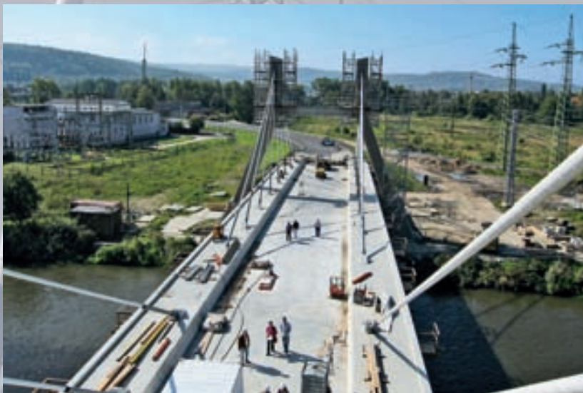
View onto the bridge deck
