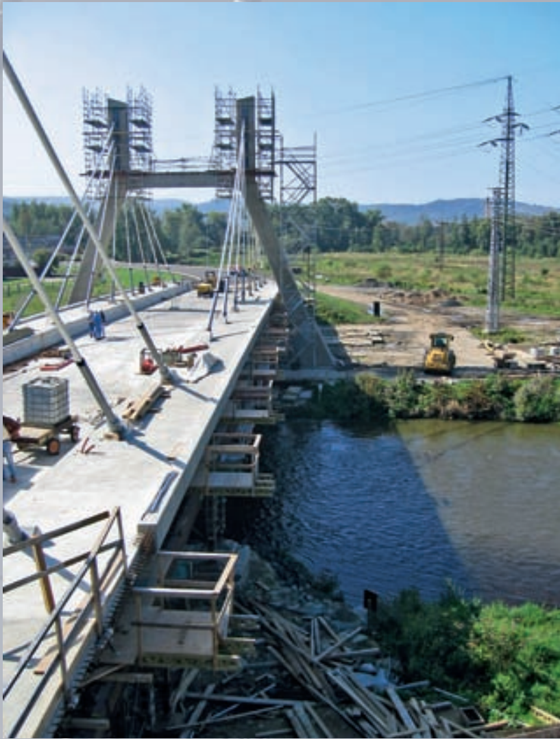
Bridge deck with anchorages
