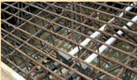
Tie Rods with Anchor Plate in Reinforcement
