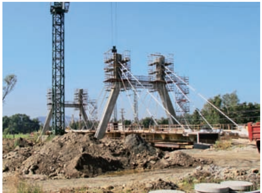
Stay Cable Bridge over Ohre River in Karlovy Vary, Czech Republic
