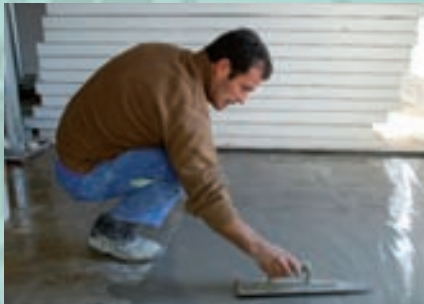
Smoothing after application of levelling paste
