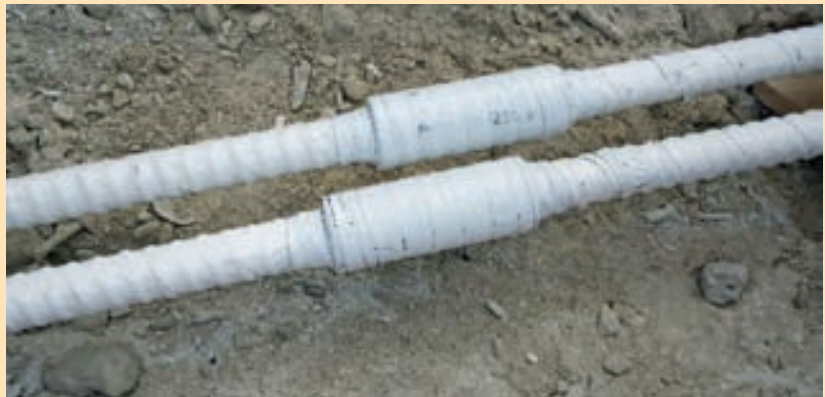
Coupler Area of Tie Rods
