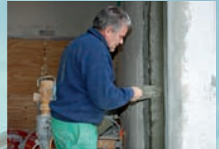
Utilization of repair mortar Fibraltchoc
