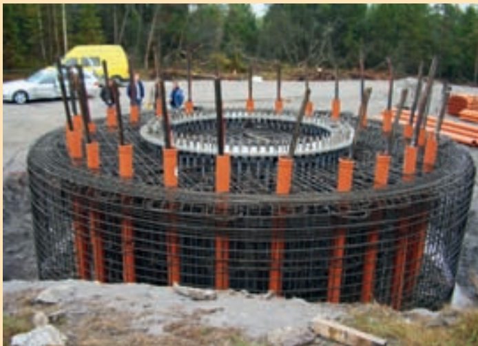
Reinforcement of foundations with SUSPA Strand Anchors
