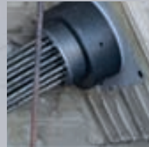
Anchorage of DYNA Grip® Stay Cables at the Pier
