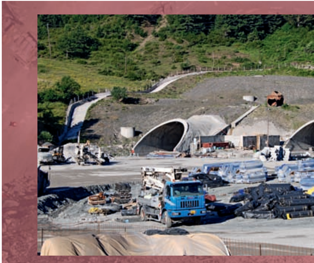
Metsovo Tunnel / Tunnel portal
