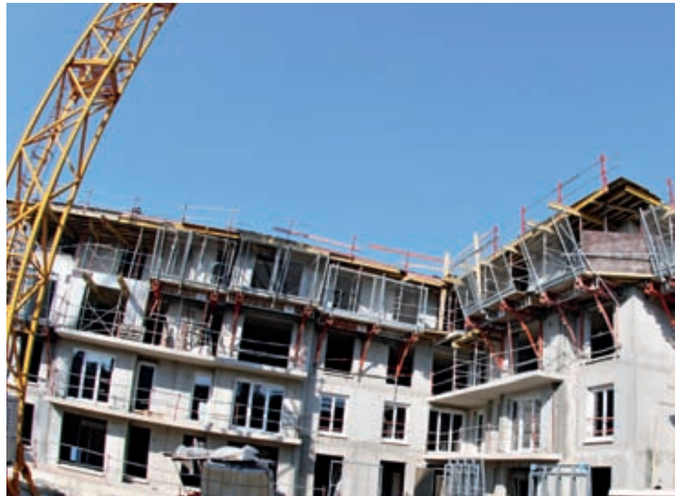
Levelling works at the facade with Finimur
