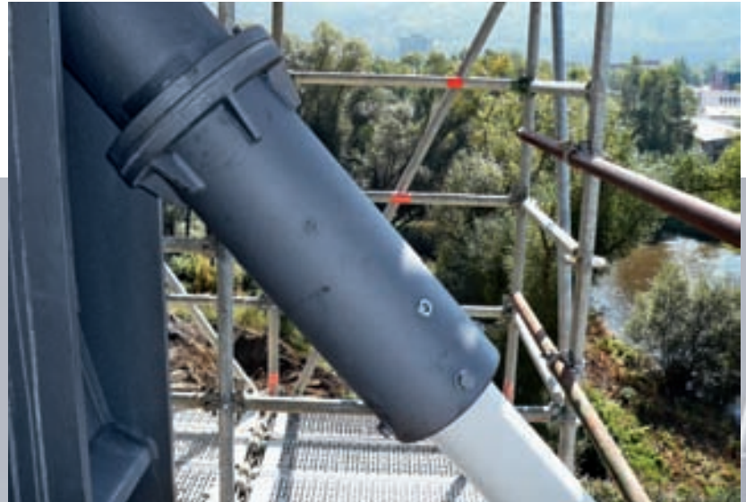
Anchorage of DYNA Grip® Stay Cables at the Pier
