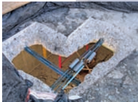
Recesses with repaired monostrands
