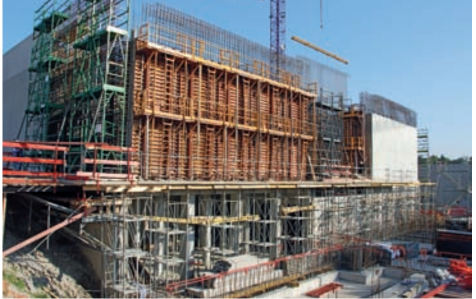
Formworking at new plant building
