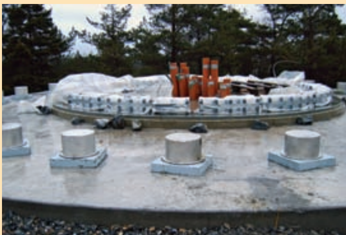
Completed foundations containing installed SUSPA Strand Anchors
