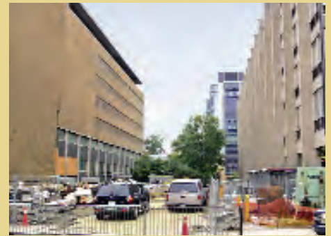
Site layout before construction
