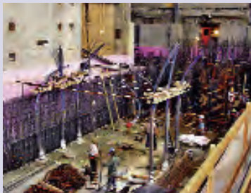
Tight space, stringent tolerances, precision execution
