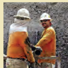
Installing the DYWIDAG Multistrand Anchors using uncoilers
