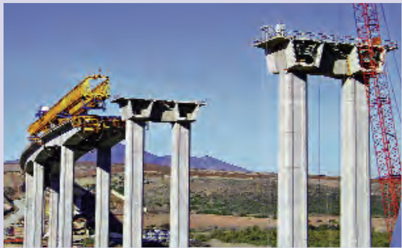
Installation of precast concrete segments using a gantry truss
