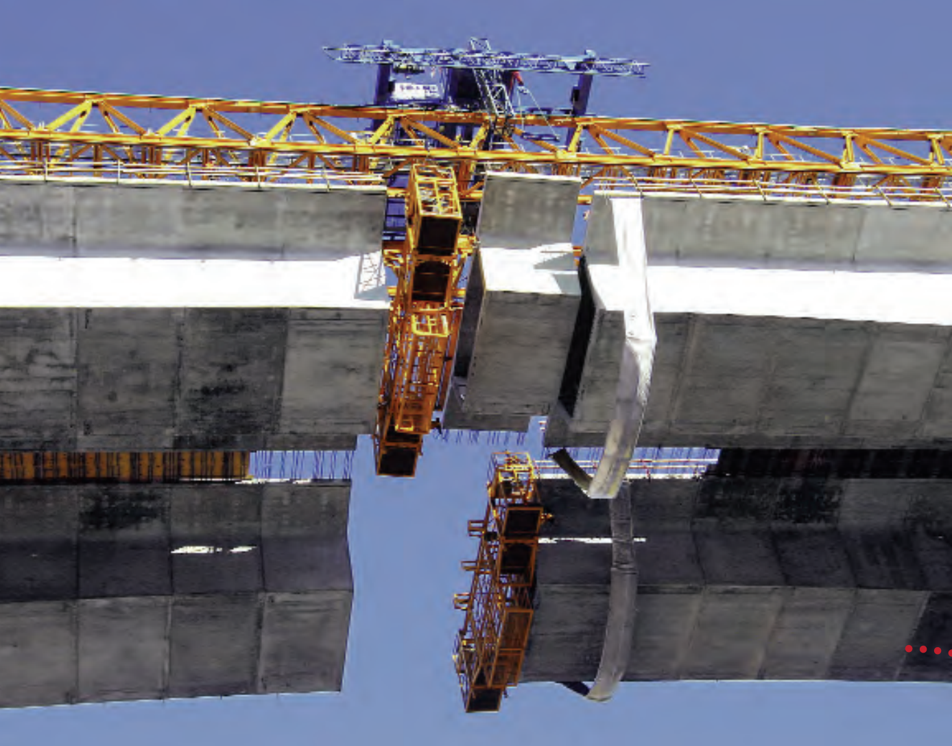
Installation of a precast concrete segment
