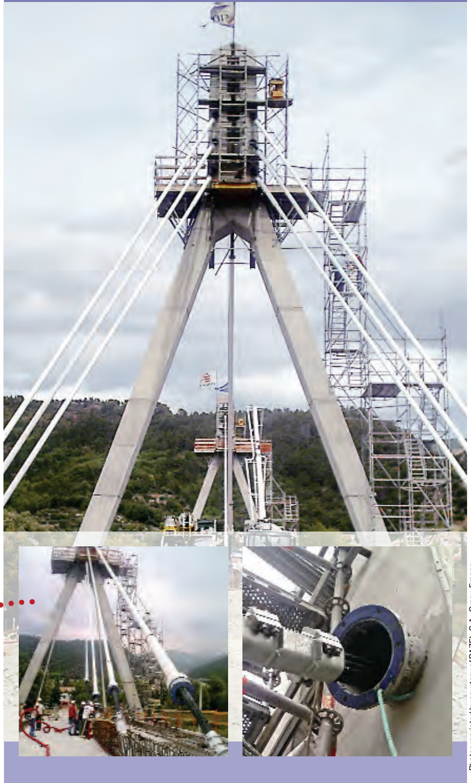
Photos reprinted by courtesy of RAZEL-S.A., Orsay, France
