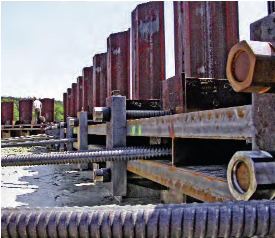
Waling bolts and tie rod connection
