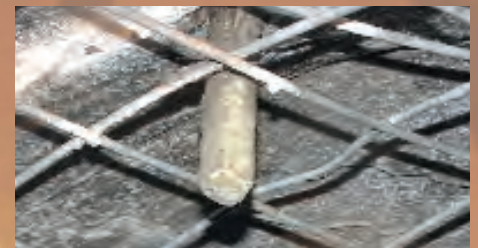
Installed DSI Fiberglass Rebar
