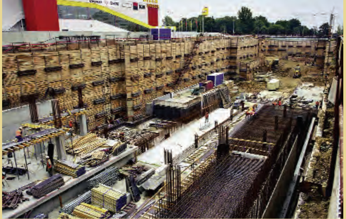
Open cut of the Prosek station
