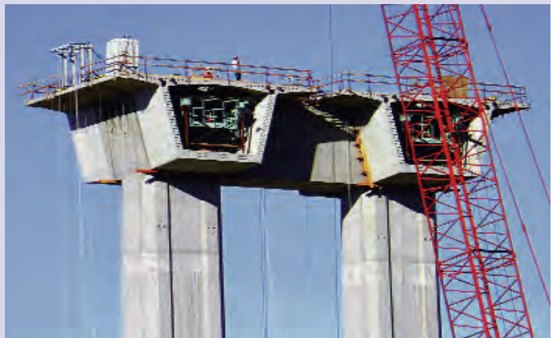
Ready concreted pier cap above a pair of piers
