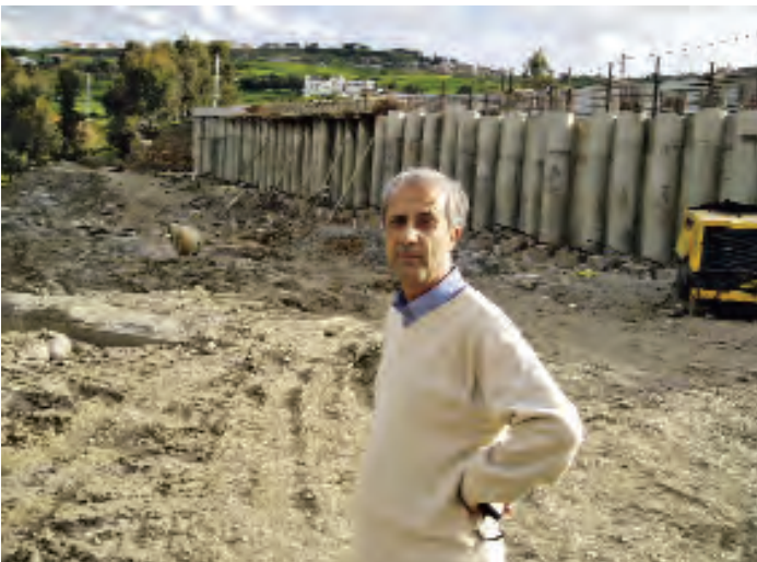
Installation of DYWIDAG Multistrand Anchors on site in Algiers
