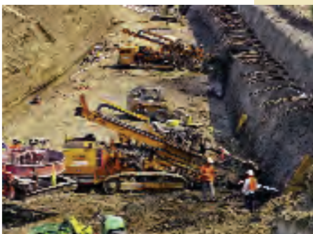
Installing the DYWIDAG Multistrand Anchors using uncoilers
