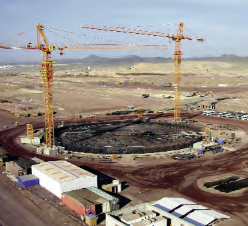
View onto construction site Bal Haf, Yemen
