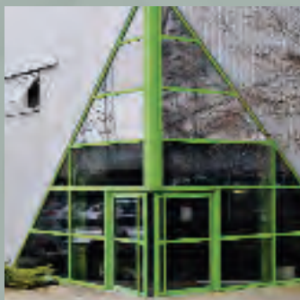
Technique Béton, office and production, Moissy Cramayel, France
