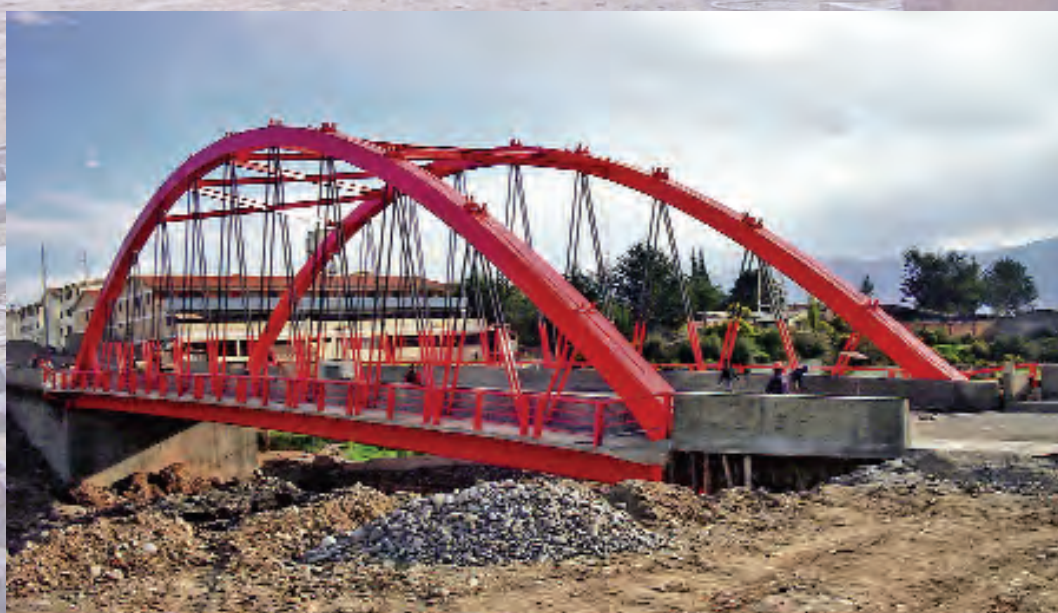
Alcides Carrión bridge in Huánuco, Peru
