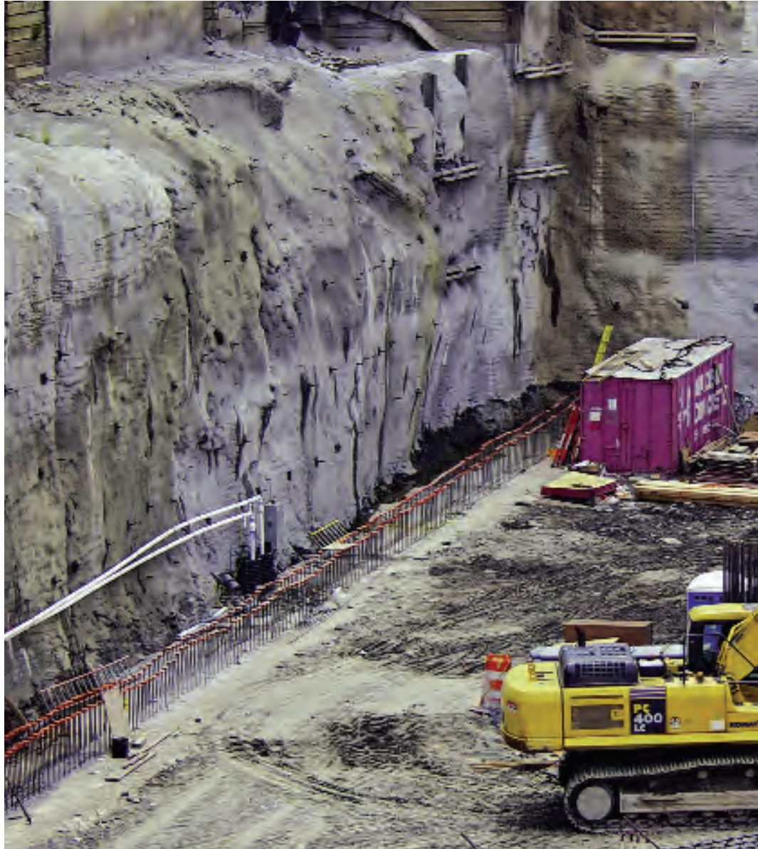
Working on the foundation slab
