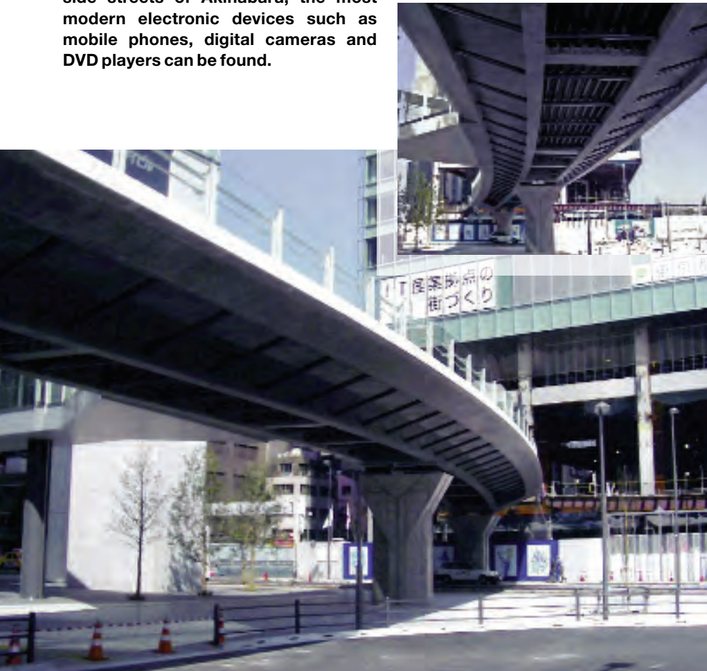
Completed pedestrian deck
