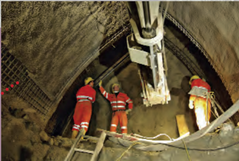
Drilling works in the sidewall drift (AT-118/DR)
