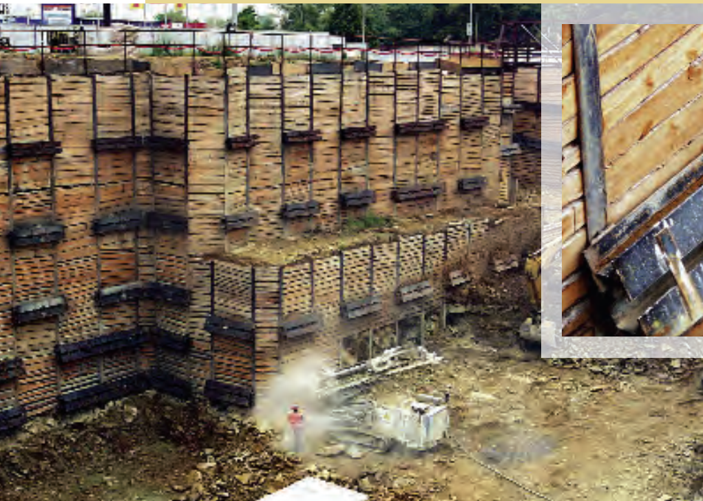
Installation of temporary DYWIDAG Multistrand Anchors
