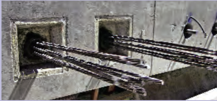
Detail view of the DYWIDAG Strand Anchors
