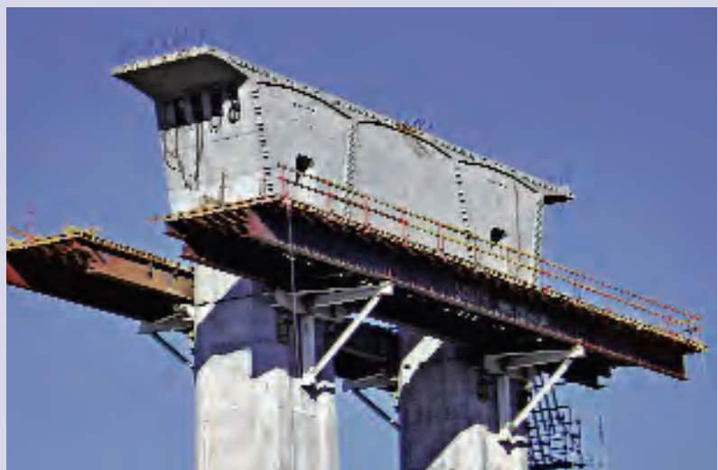
Precast concrete segments installed in a pair of piers
