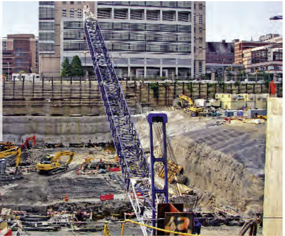
Excavation including retaining walls
