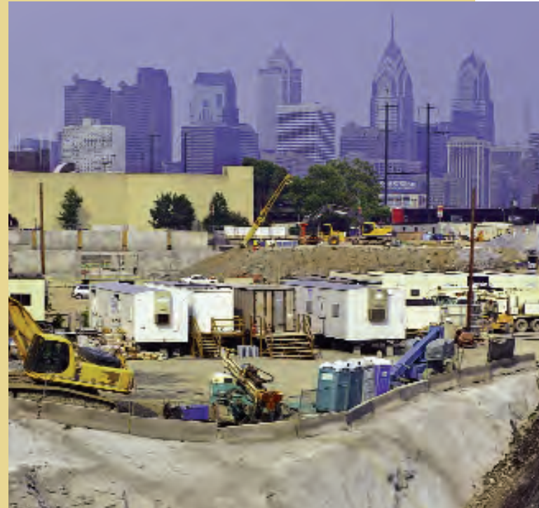
Overview of the excavation
