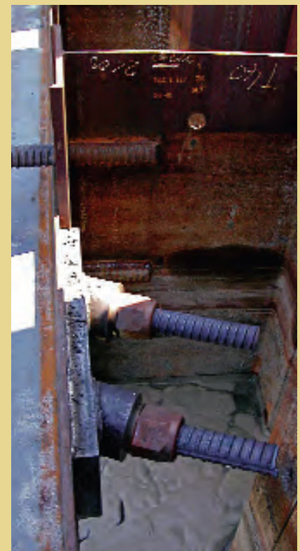
Waling bolts and tie rod connection
